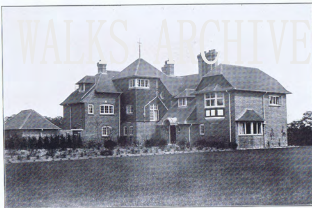
"THE PATCH," HOOK HEATH, WOKING. Built of red bricks and roofed with red sand-faced tiles, with motor house, &c., on the north side. The house stands on the ridge overlooking the valley of the Wey.
