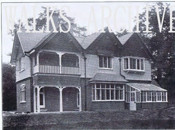
"HILLSIDE," CHURCH HILL ESTATE, HORSELL. Red bricks and white rough cast, red tiled roof and lead glazing.
